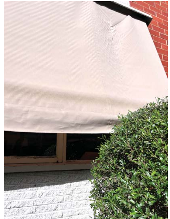
External sunblinds protect windows from the heat
