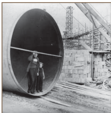
Christine and her mum alongside engineering works at the Snowy Mountains Hydroelectric Scheme, 1953
